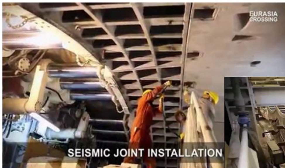
The Eurasia Undersea Tunnel Project
